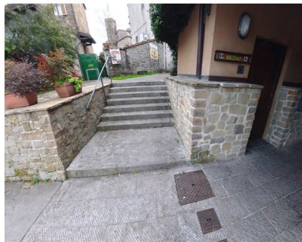
7 Accessible toilets in the Via Soccorso car park and adjacent staircase that connects to the village entrance
