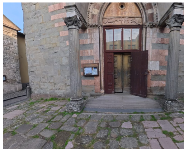
20 Second ramp to access the entrance of the Church
